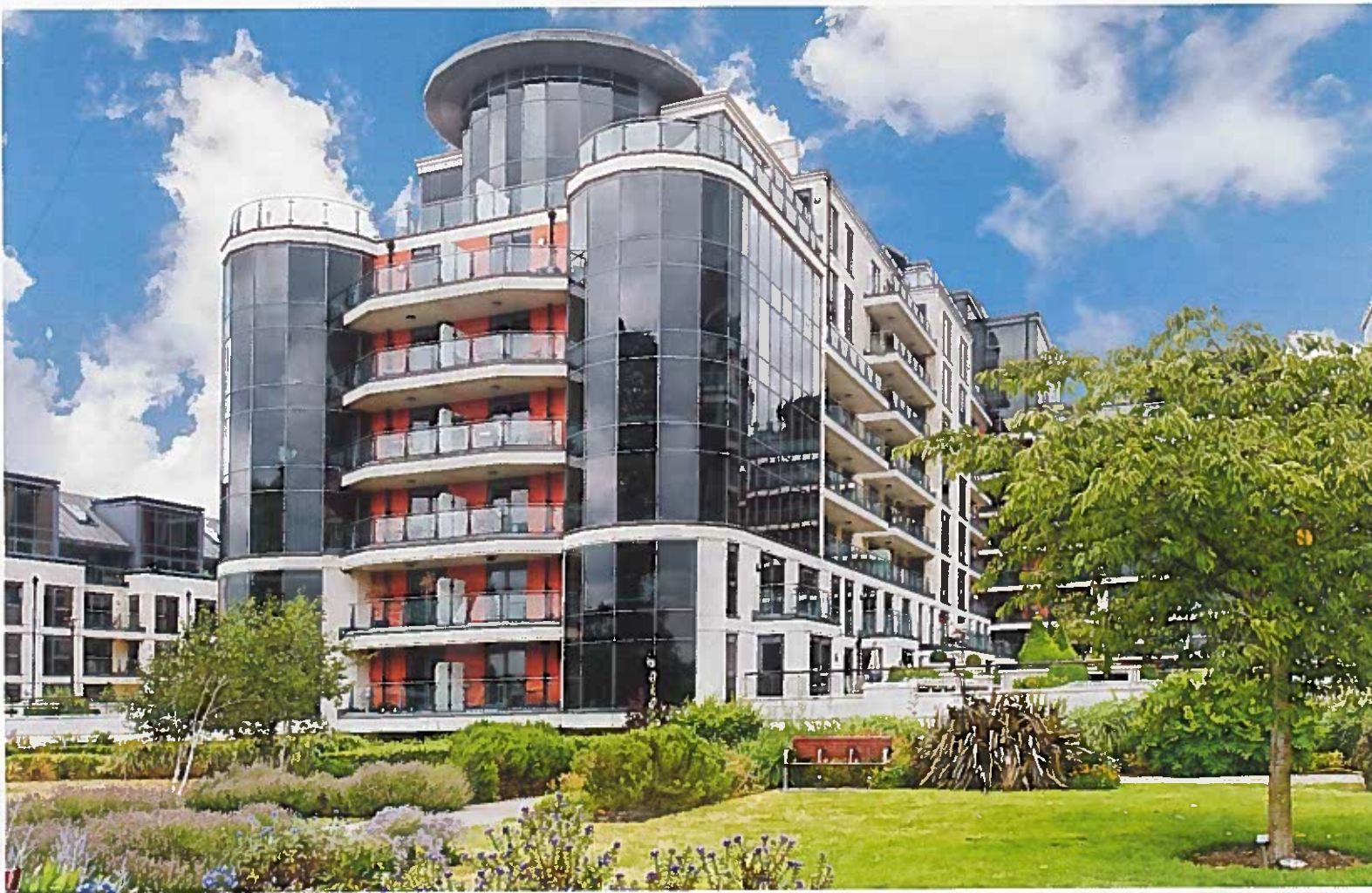
From top: the six-bedroom penthouse at The Tower, Chelsea Creek, London, £16.95m. Neighbouring Dolphin House, where a two-bedroom flat is available for £3m. Both through Knight Frank
